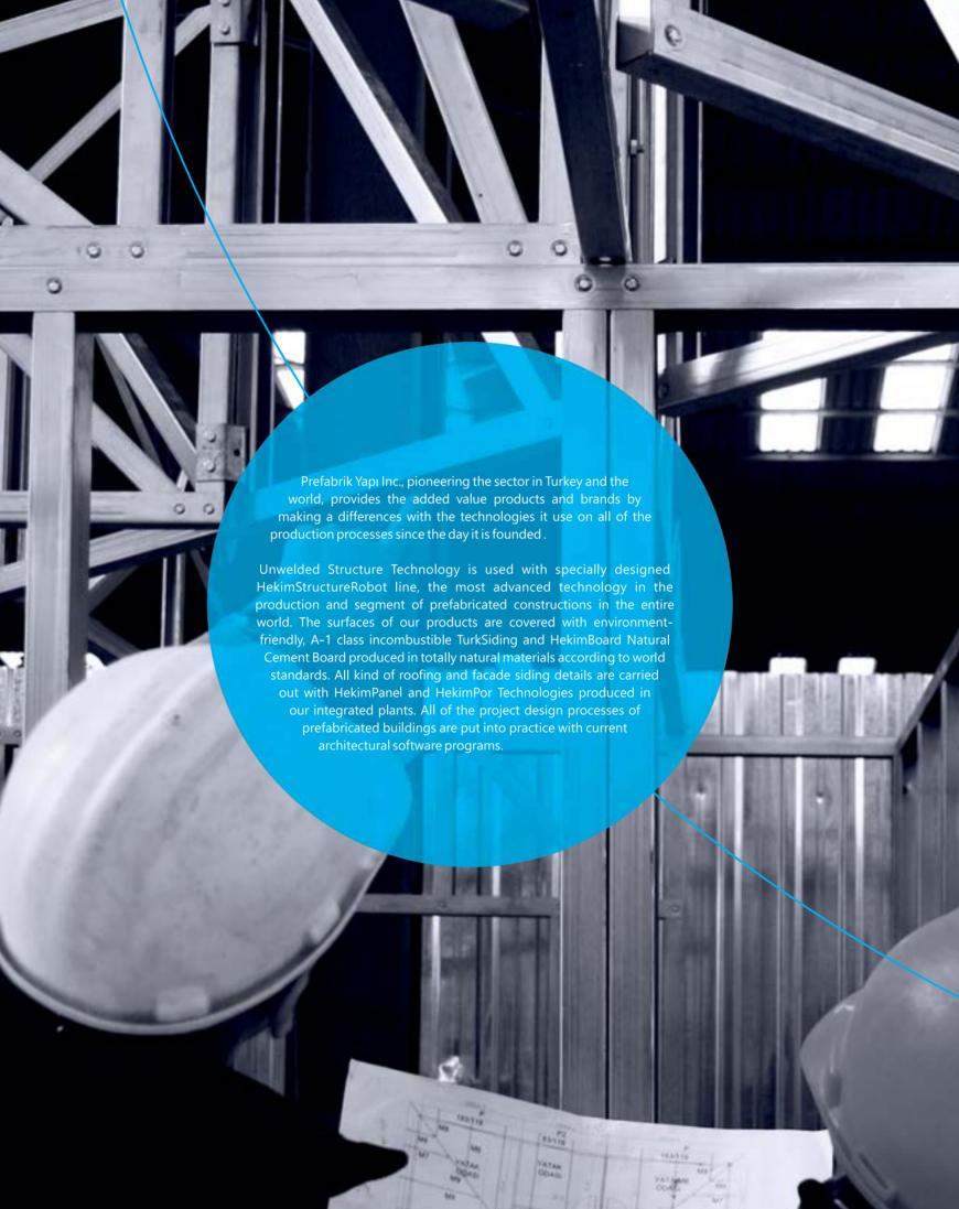
All of the construction elements are produced by cold-forming of galvanized steel through specially designed weldless construction technology. Walls, frame, roof, truss and other building components of the building designed in the project design process are created by connecting profiles with bolts and nuts which produced in HekimStructureRobot lines.
